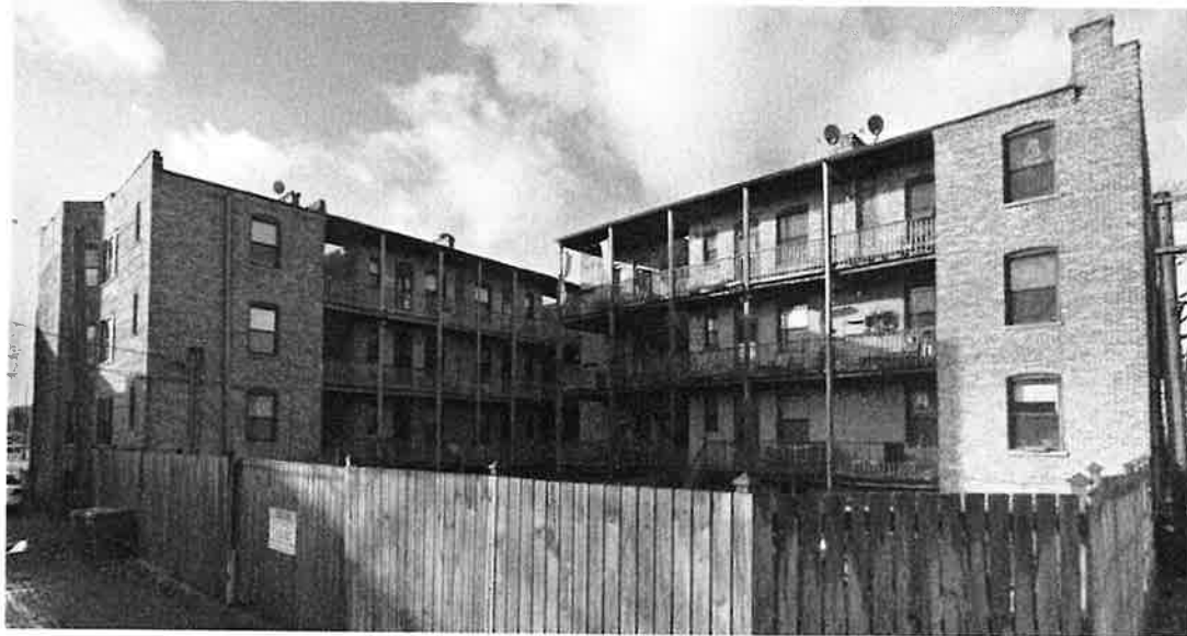
South and East Views of Building (Source: Google Maps)
