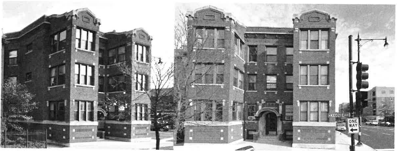
Northwest and West Façade Views of the Building (Source: Google Maps)
