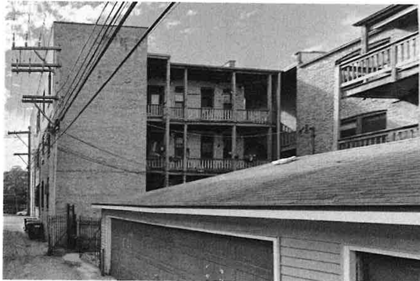
South, Southeast and Northeast Façade Views of the Building (Source: Google Maps)
