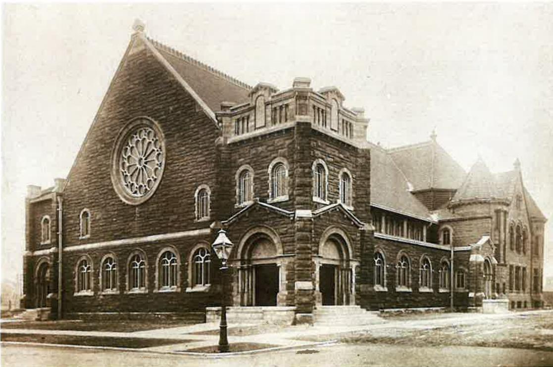
Below: Photograph of the church circa 1906. The 1896 building is still present at the rear. (Source: Hyde Park Union Church archives)
