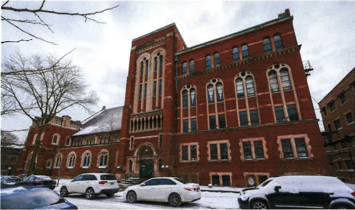
Above: The north elevation of Hyde Park Union Church. The Education Wing begins at the middle tower and extends westward to the alley.
