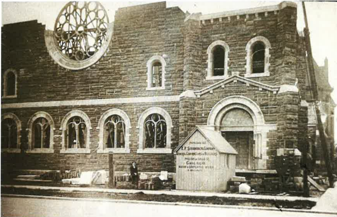
Above: Glass plate photograph of the church façade during construction, circa 1904-05. (Source: Hyde Park Union Church archives)
