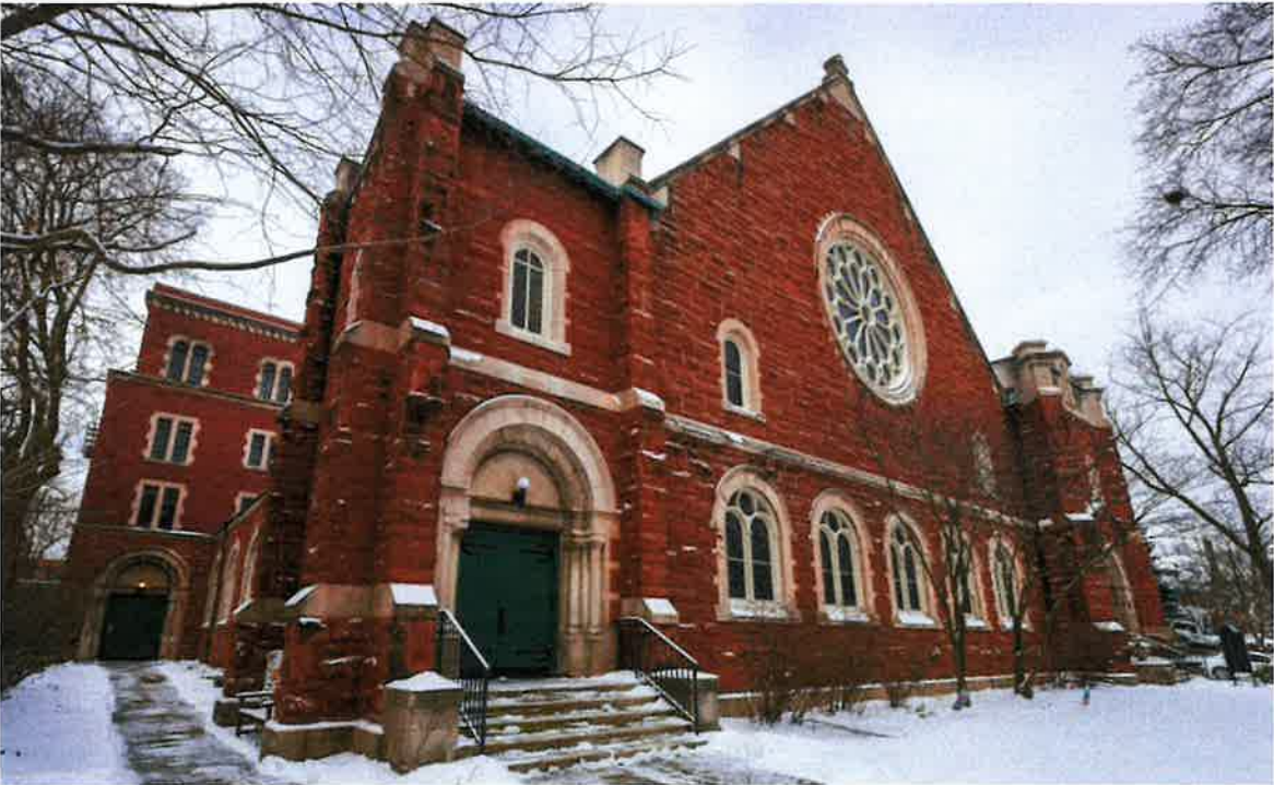
Below: Looking NW at the east elevation of Hyde Park Union Church. At left is the recessed portion of the building which gives a clear view of the Education Wing. (Photos by Patrick Pyszka)
