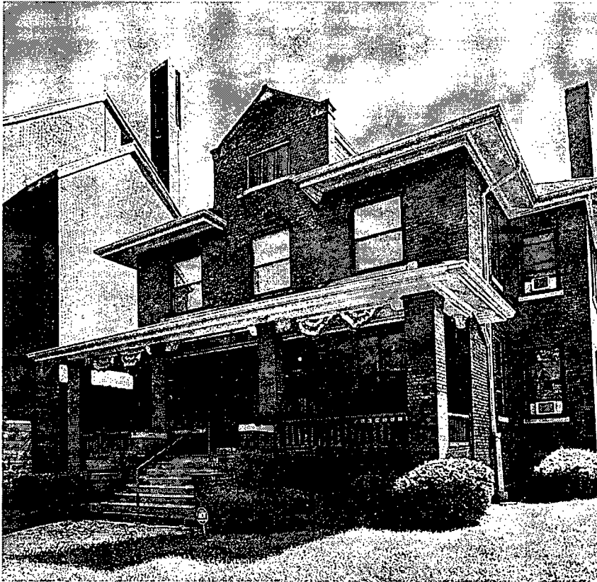
Pictured above is the former Holy Rosary Church rectory now used as church offices for Greater Tabernacle Cathedral. In contrast to Beman's church design, the design of the rectory is modest and absent of applied architectural detailing.
