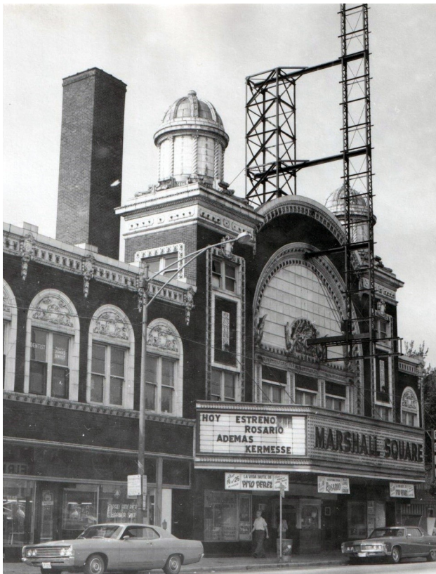
By 1972, the neon Marshall Square blade sign had been removed leaving the armature. Source: Theater Historical Society of America.
