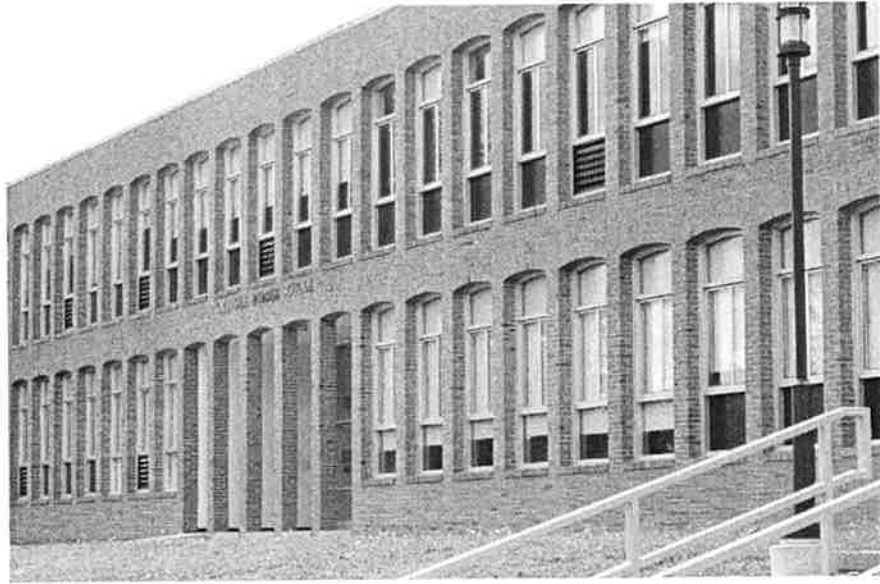
At the Northside Junior High School in Columbus, Indiana (1961), Ben Weese used a traditional system of brick arches and piers.
