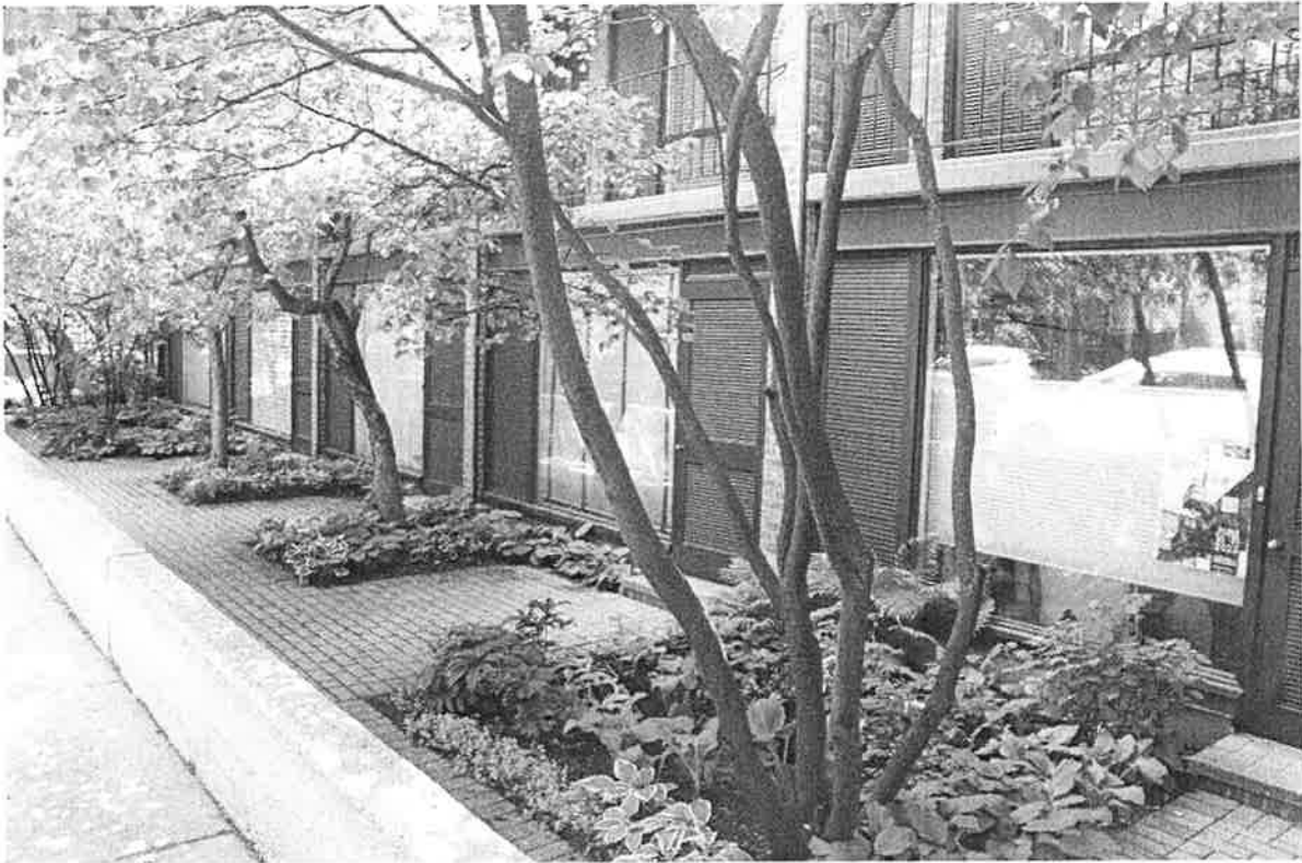
The ground floor is recessed below grade with a landscaped front garden. Louvered entrance doors to each apartment are located on the exterior, eliminating the need for internal corridors and clearly conveying the building's residential function.
