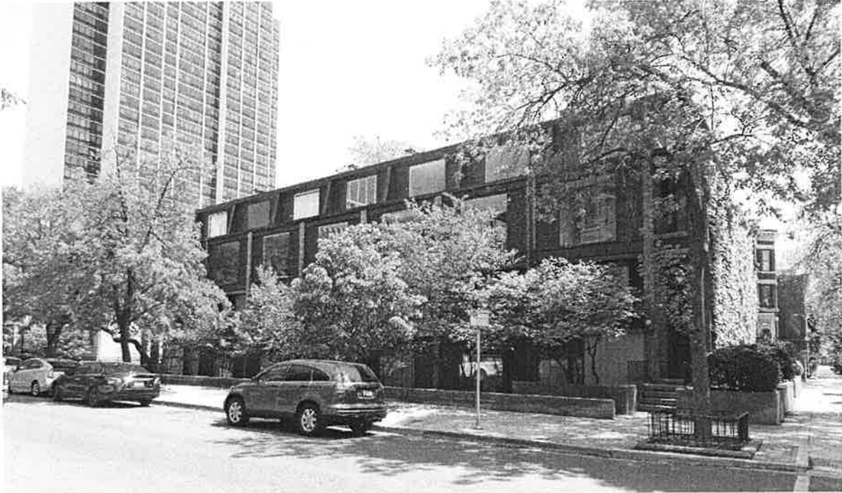
The front elevation of the Eugenie Lane Apartments. Chicago common-brick piers divide the façade into 7 bays. The recessed mansard roofline reduces the building's apparent height.
