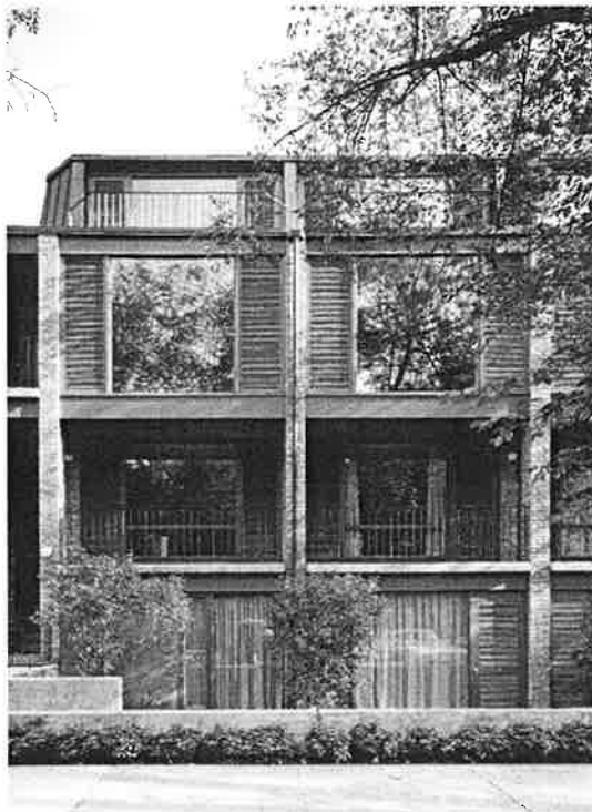
The exterior wall at the second floor is recessed creating a gallery which provides access to the apartments. Source: Hedrich Blessing, 1962, Chicago History Museum, HB-25565.
