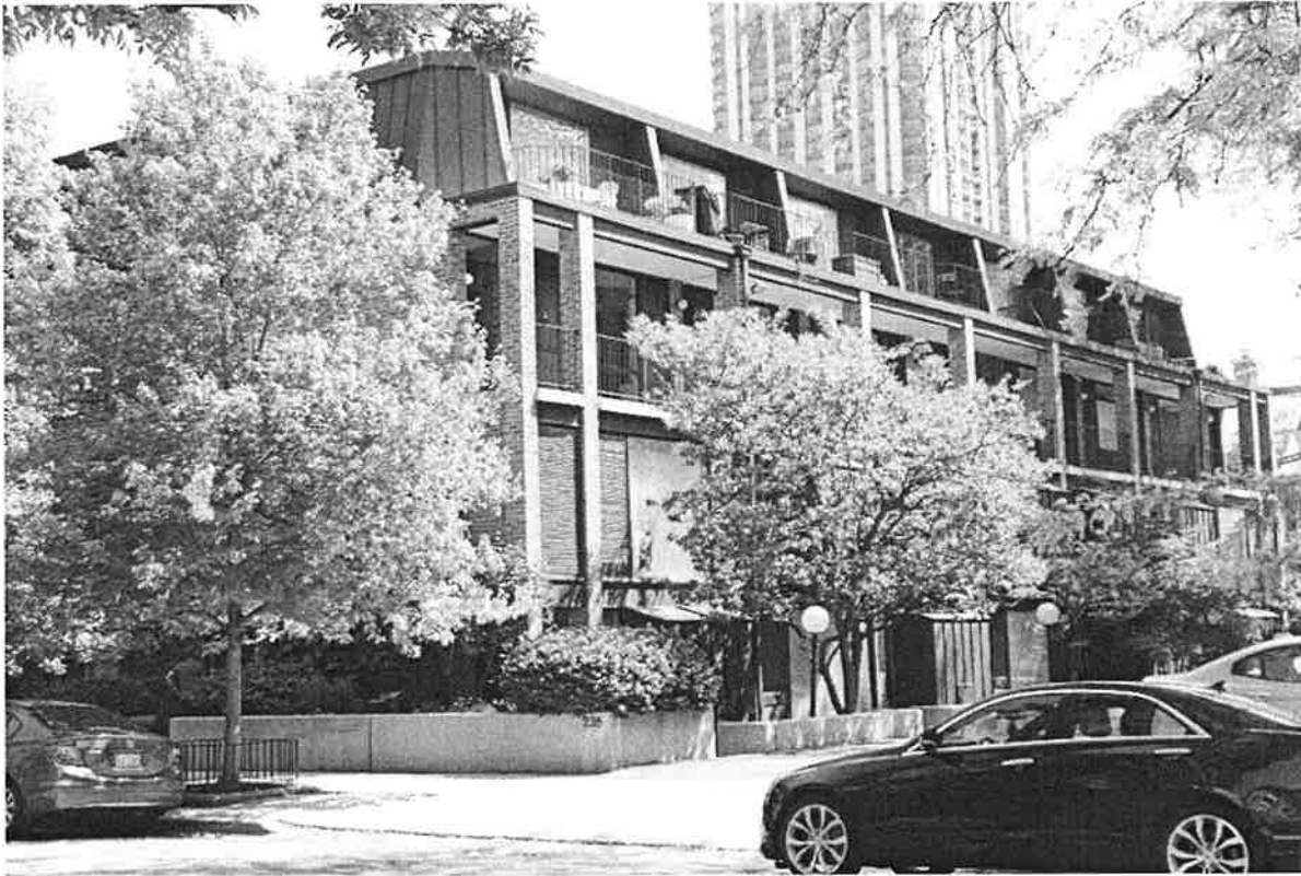
The rear elevation with projecting bays clad in standing-seam sheet metal that contain closets.
