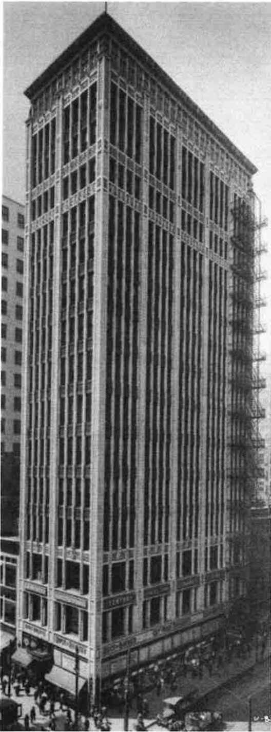
Left: The Century Building ca. 1920.
