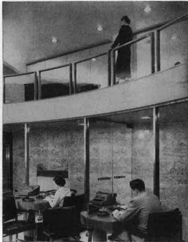
ENDURO and glass separate lobby and banking floor, act as balcony rail and draft screen.
