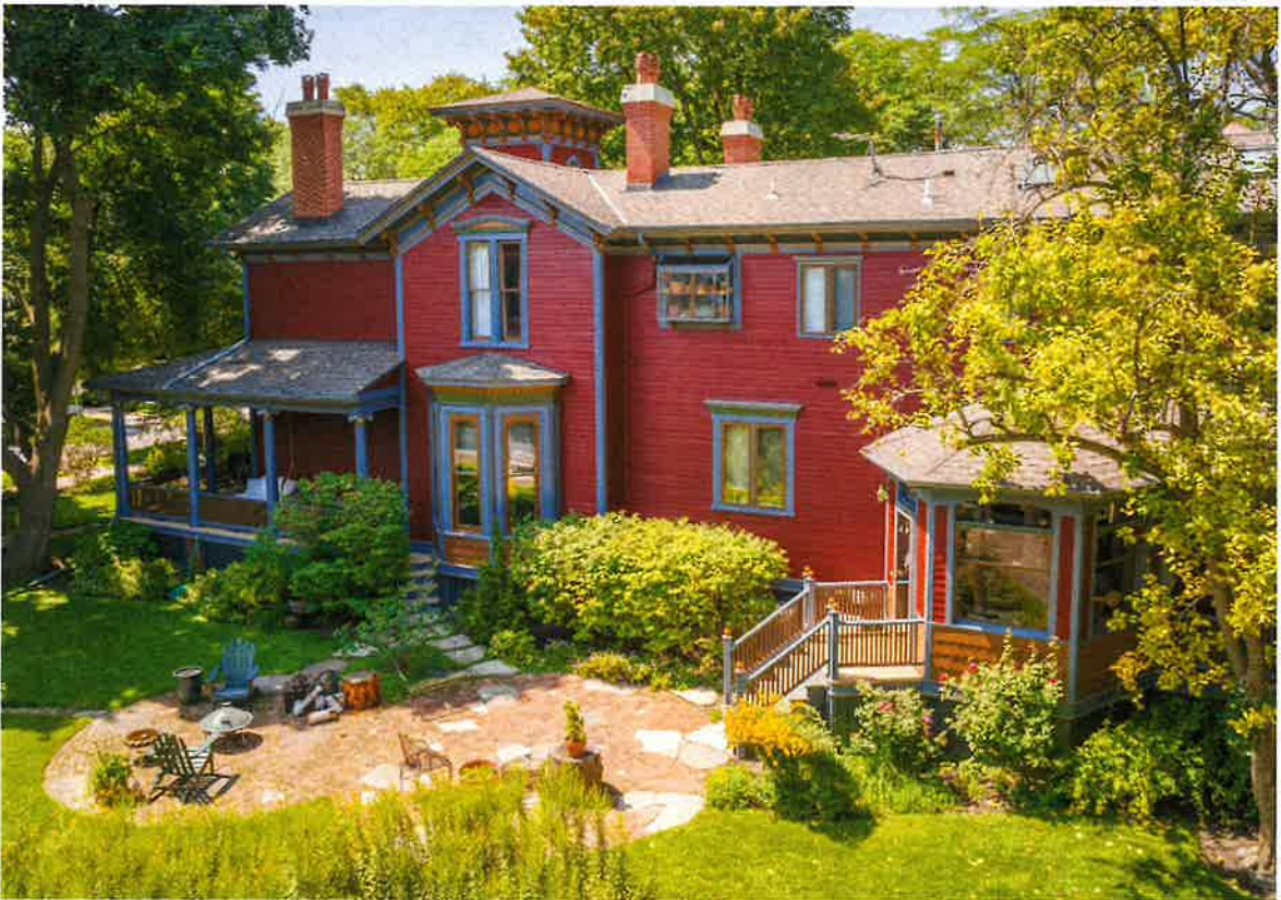
Top Photo: South Elevation, wood trim detailing Bottom Photo: East Elevation, including a later 1-story rear addition. The farmhouse's original rear wall was immediately south of the pictured addition. Source: Troy Walsh, Drone Media Chicago (2023)
